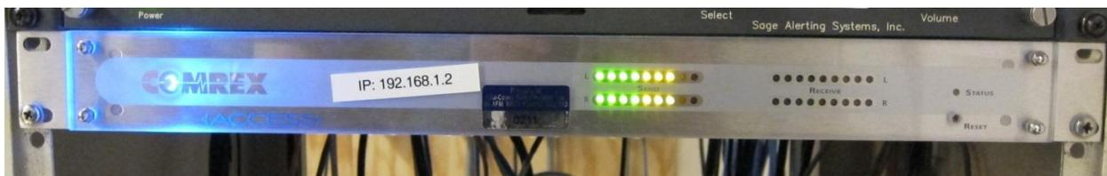
*Comrex Rack-Mount Unit Face shown in normal static state without a link to the remote unit.*
